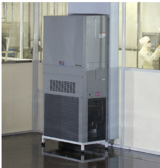
A/C Module mounted to return plenum, with cooled air ducted to fan/filter unit.
