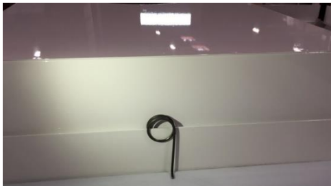
Figure 3: 1-Arm Ceiling Clip holds down a ceiling panel with a FFU installed on the opposite side of the joist.
