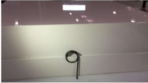
Figure 3: 1-Arm Ceiling Clip holds down a ceiling panel with a FFU installed on the opposite side of the joist.
