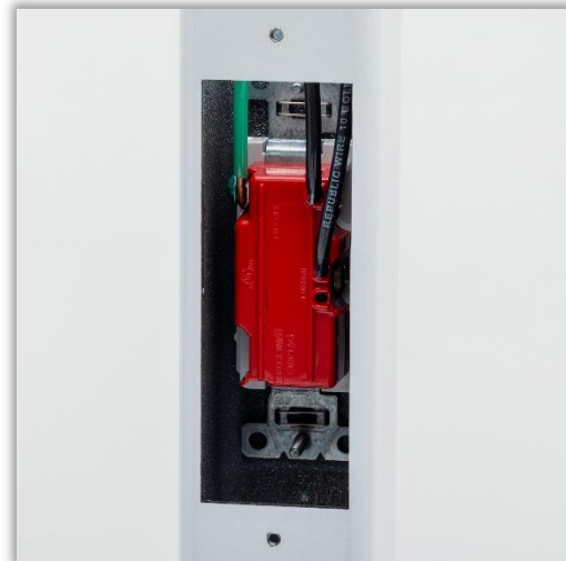
Figure D: Switch Back (cover plate removed)
