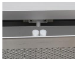
Photo 1: Friction catches hold the screen to the fan module housing.
