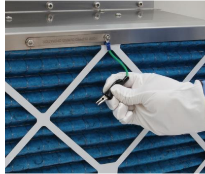
Photo 5: Clipping the grounding wire to metal threads in the pre-filter.
