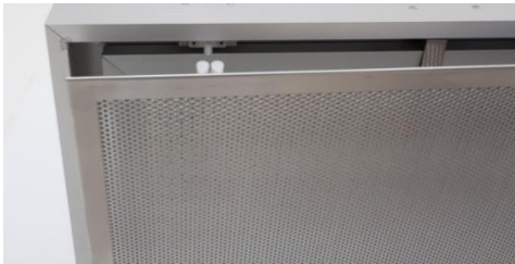
Photo 1: Friction catches hold the outer screen to the fan module housing.
