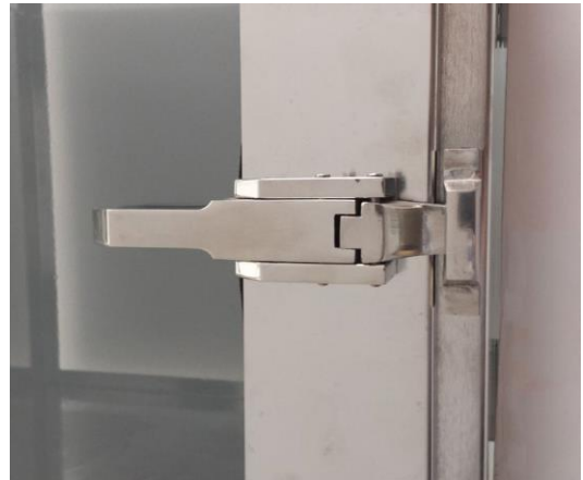
Figure 9: Properly aligned LiftLatch
