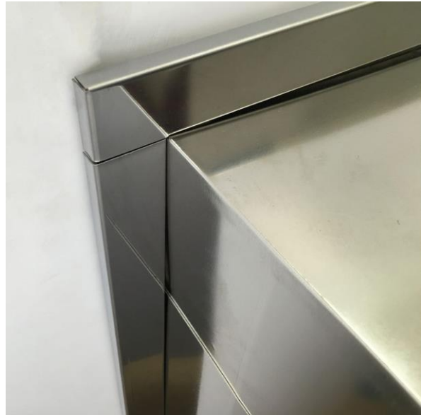
Figure 8: Snap the bracket covers back into place to hide the lag bolts and other hardware
