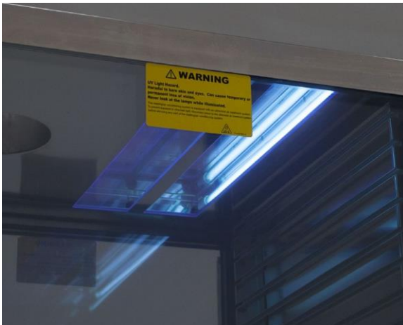
Figure 13: Recessed UV-C light
