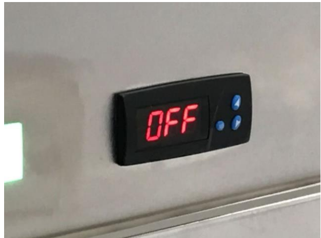
Figure 14: Cycle time can be adjusted via the timer on the “dirty”-side of the pass-through
