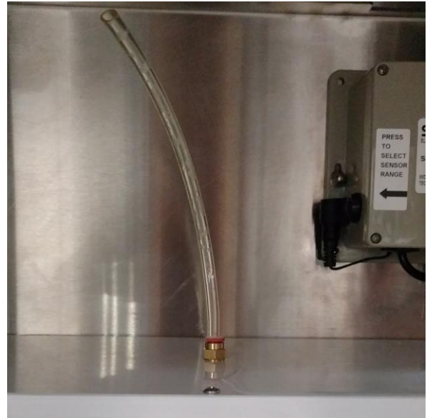
Figure 6. Air relief valve on top of the waste water tank
