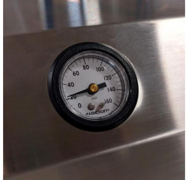
Figure 2. Pressure gauge shown with an empty water tank, reading only the pressure in the diaphragm (25 psi standard from factory)
