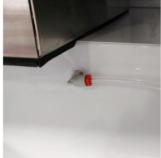
Figure 5. FFU push-to-connect fitting for pressure gauge
