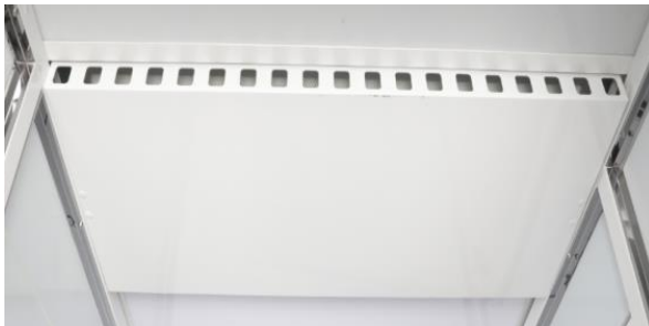
Figure 1: White caps must be removed to expose the screws that hold the outer screen to the fan module housing.
