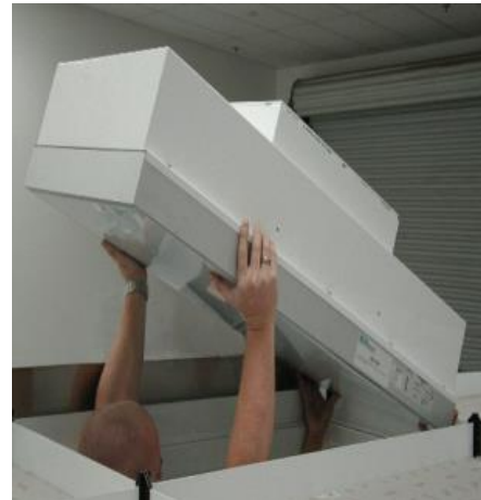
Figure 14: FFU pushed up on one side for removal
