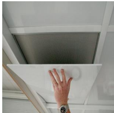
Figure 12: Panel attaching to exposed HEPA filter
