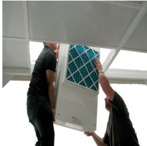
Figure 16: FFU rotated 90° and lowered completely from ceiling grid
