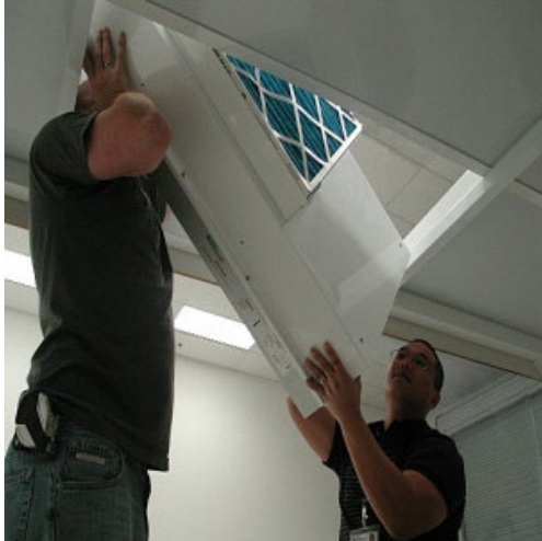
Figure 15: Personnel rotating FFU to remove from ceiling grid
