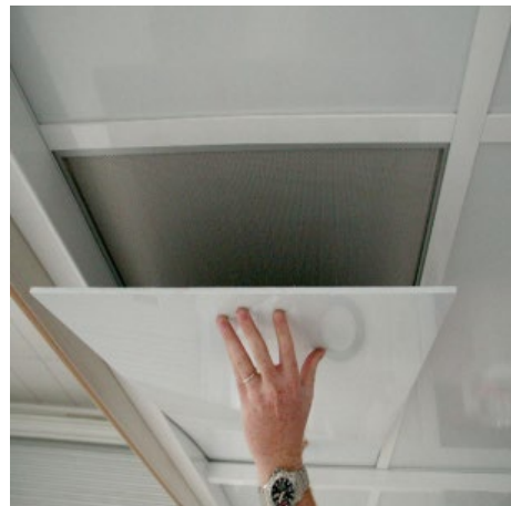
Figure 12: Panel attaching to exposed HEPA filter
