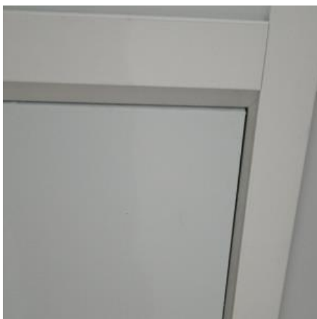
Figure 10: Panel fully attached to filter screen without overlapping edges
