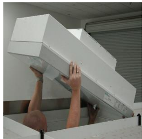
Figure 11: FFU pushed up on one side for removal
