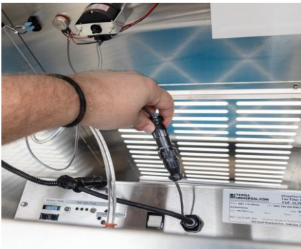
Figure 24: Reconnecting cables after panel reinstall
