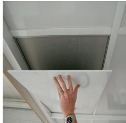
Figure 9: Panel attaching to exposed HEPA filter
