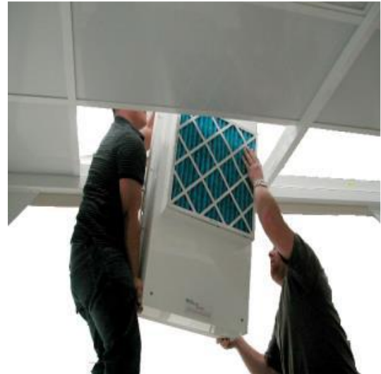
Figure 13: FFU rotated 90° and lowered completely from ceiling grid
