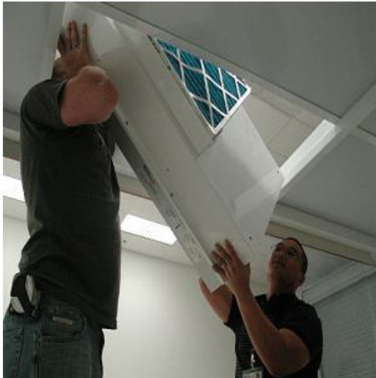
Figure 12: Personnel rotating FFU to remove from ceiling grid
