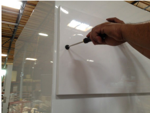
Photo 26: Outside access panel door shown while fasteners are being removed
