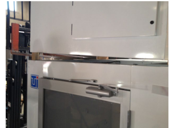
Photo 12: Wood stud removed and Blower Module is being supported by one of the four (4) 2"x4" wood blocks
