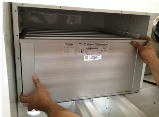
Photo 30: HEPA filter shown being removed
