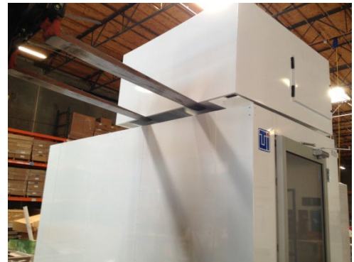
Photo 15: Forklift lowered and Blower Module shown with two (2) of the 2"x4" wood blocks removed
