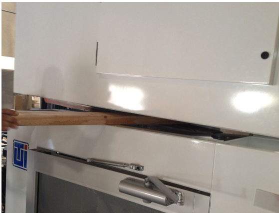
Photo 11: 2"x4" wood stud being removed from underneath the Blower Module
