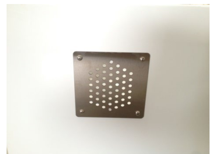
Photo 6: Make-up air vent
