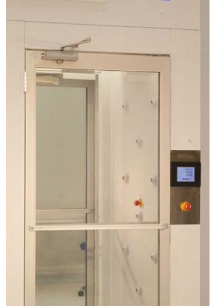
Photo 24: Emergency Stop Buttons – one (1) located inside and one (1) located outside the unit
