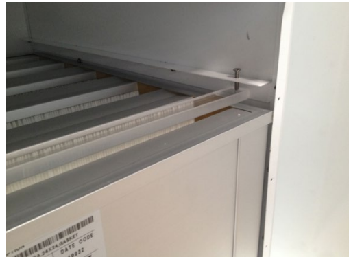
Photo 29: HEPA filter shown held in place by a polycarbonate shim
