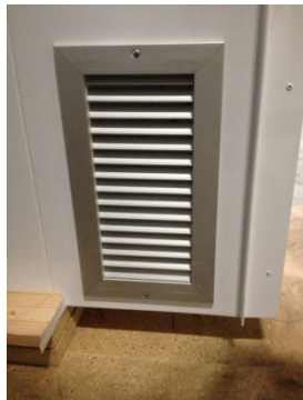
Photo 2: Removable corner vent at each corner inside the Air Shower/Tunnel
