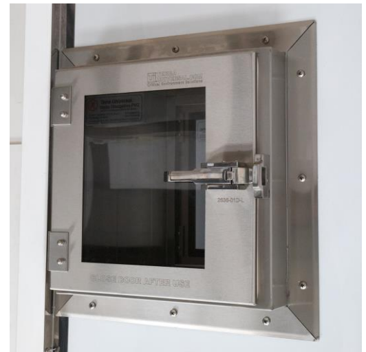
Figure 8: Pass-through with standard mounting brackets, fastened to the wall
