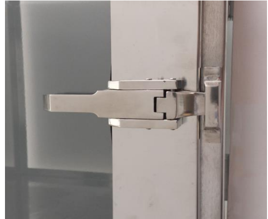
Figure 15: Properly aligned LiftLatch
