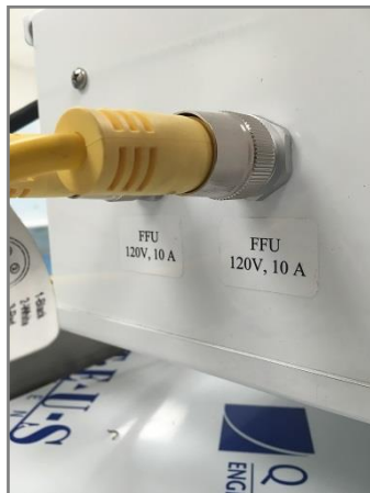
Figure 3: PDM connections for the fan/filter units
