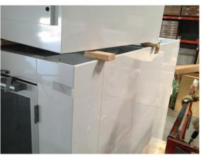
Photo 10: Blower Module shown positioned on the 2"x4 wood blocks at two (2) of the corners
