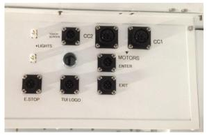
Photo 17: Main Junction Box Connections Panel
