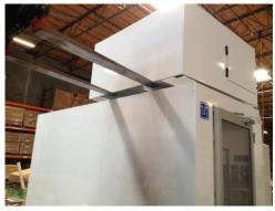
**Photo 15:** Forklift lowered and Blower Module shown with two (2) of the 2"x4" wood blocks removed
