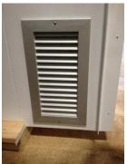
Photo 2: Removable corner vent at each corner inside the Air Shower/Tunnel
