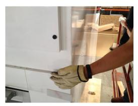
**Photo 16:** Blower Module shown manually pushed into place
