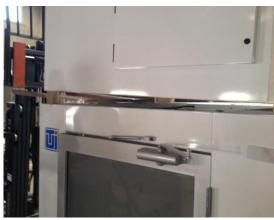
Photo 12: Wood stud removed and Blower Module is being supported by one of the four (4) 2"x4" wood blocks
