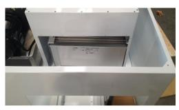
Photo 30: HEPA filter shown being removed
