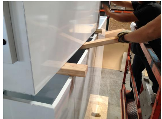
Photo 13: 2"x4" wood stud used to lever the Blower Module up to remove the two (2) 2"x4" wood blocks
