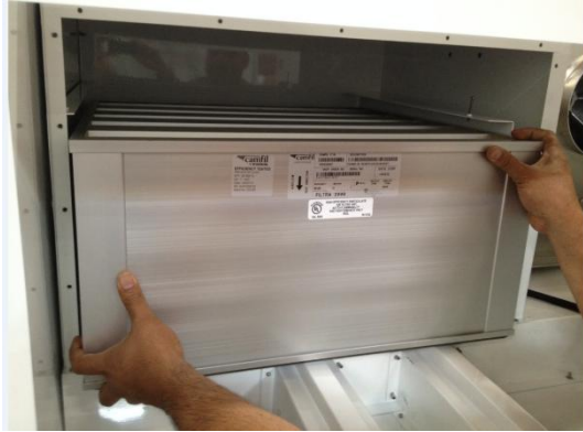
Photo 30: HEPA filter shown being removed
