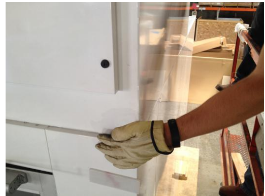
Photo 16: Blower Module shown manually pushed into place
