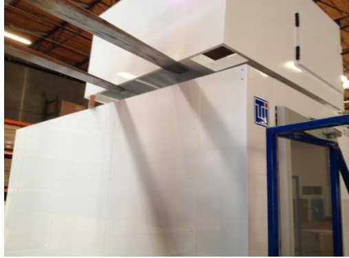
Photo 14: Forklift shown levering the Blower Module to enable removal of the 2"x4" wood blocks
