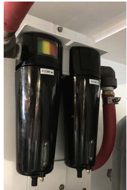
Figure 8. Two-Stage Coalescing Filtration
