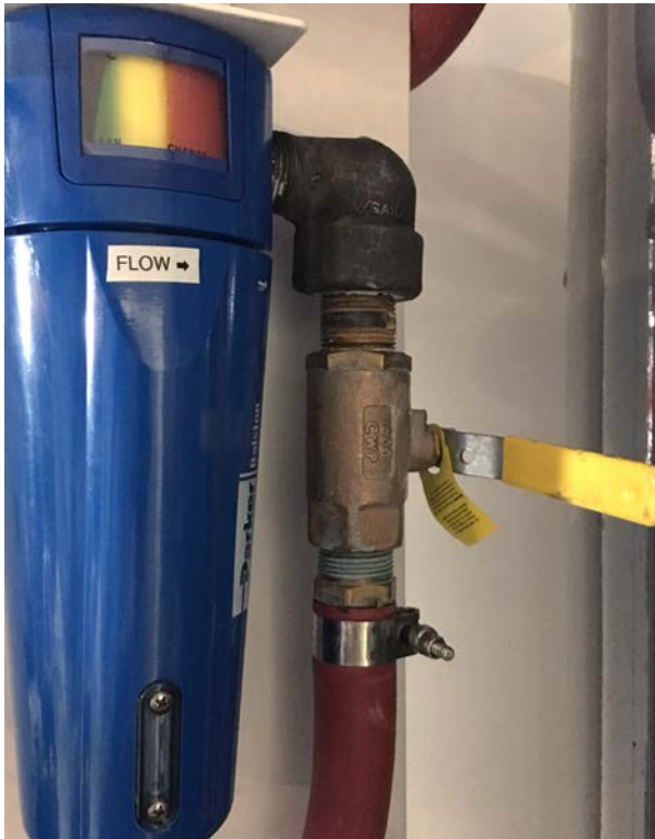
Figure 2. Post-Filter Shutoff Valve (shown in "closed" position)
