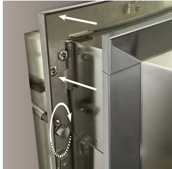
Figure 12: Snap the bracket covers back into place to hide the lag bolts and other hardware
