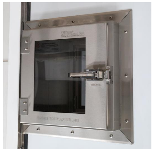
Figure 6: Pass-through with standard mounting brackets, fastened to the wall
