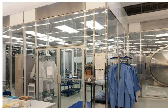
Hardwall modular cleanroom made of static-dissipative PVC for an academic research institution studying microsatellite technology.
