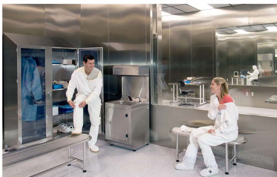
BioSafe modular cleanroom made of 304-grade stainless steel for GMP-grade pharmaceutical manufacturing and packaging.
