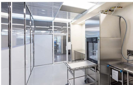
Hardwall modular cleanroom made of polycarbonate with an opaque, polypropylene modesty panel for medical device manufacturing.
