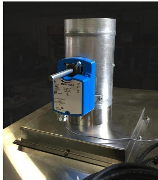
Figure 2. Electric Damper (square filter inside base)
