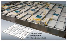
Powder-coated steel grid supports standard 24" x 48" fan/filter units, lights, or ceiling panels
