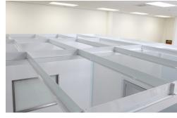
Room-Side Replaceable Fan/Filter Unit: Available with HEPA and ULPA filters.
