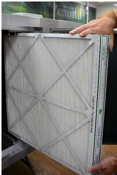
Insert Post Filter into Tracks
