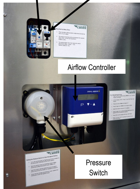
24VAC Breaker Switch Start-Up Delay Timer
