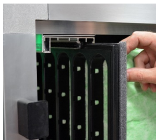
1 Install Filter into Tracks
