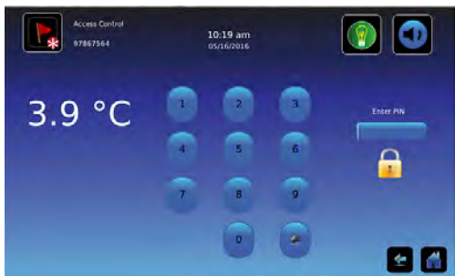
Access Control keypad
