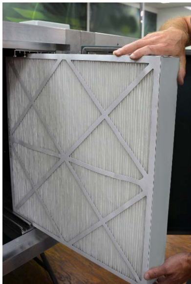
Insert Post Filter into Tracks
