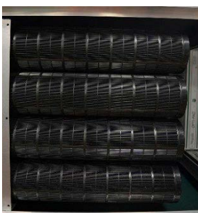
Cylinder Filters Installed
