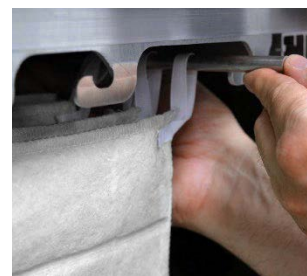
Place Support Rod on Hanging Supports
