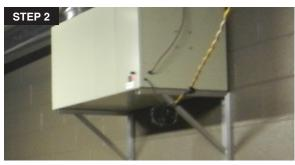
2. **Secure the unit to the wall OR ceiling**, using suitable supports, wall plugs and screws (not included). Make sure you have a power outlet nearby to plug the unit into.
