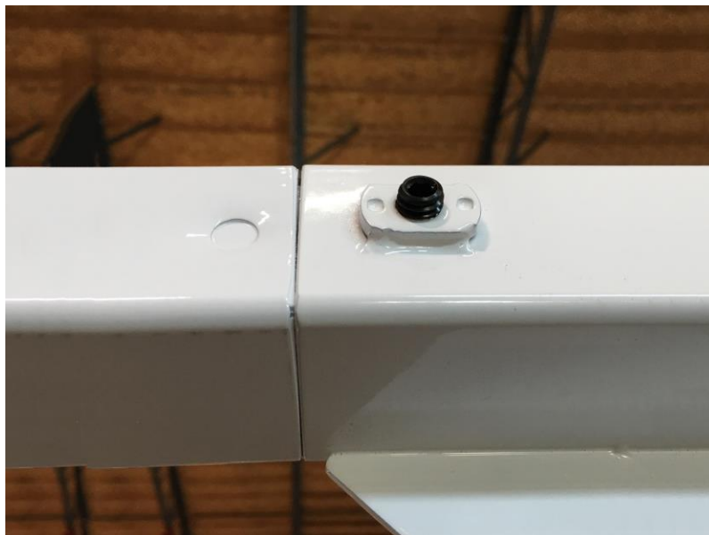
Figure 3: Use the Allen-head set screws to hold the frame members together
