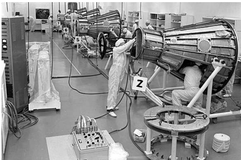
Figure 5. In the 1950s, cleanrooms became increasingly important for a variety of industries, including aerospace and electronics. Application in nuclear science also prompted the development of the first patented cleanroom system based on HEPA filtration, by Sandia Labs. Here, Mercury spacecraft are built in a cleanroom environment.
