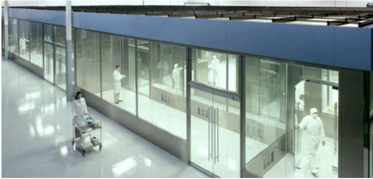
Figures 7. Modular cleanroom: this version is a multi-zone BioSafe room made of stainless steel and static-dissipative PVC. Designed to fit in existing warehouse or manufacturing space, modular cleanrooms allow development of just the right cleanroom capabilities to meet specific process needs. They can be easily expanded as production increases.
